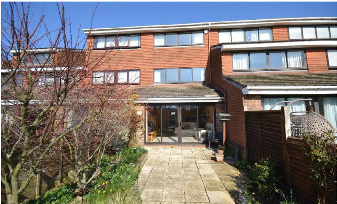
02 Rear south facing view of the property
