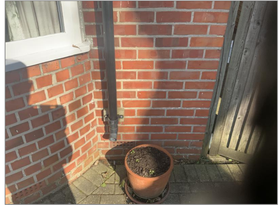
Photo - 19 Bay downpipe discharges here
