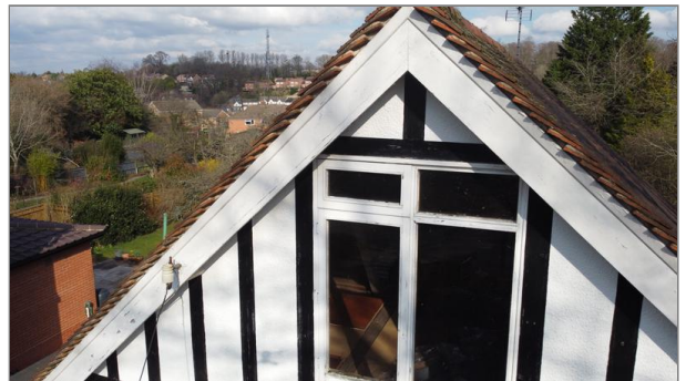
Photo - 11 Barge boards
