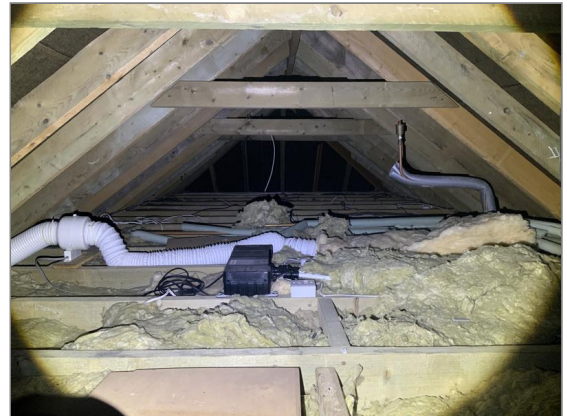
Photo - 43 To extension
