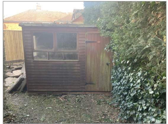
Photo - 82 Rear shed
