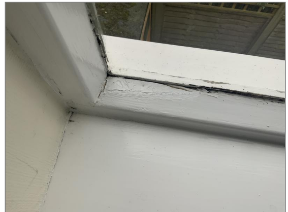
Photo - 32 Decay repair
