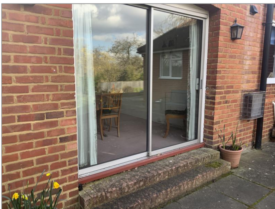
Photo - 38 Sliding doors
