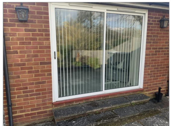
Photo - 39 Rear doors
