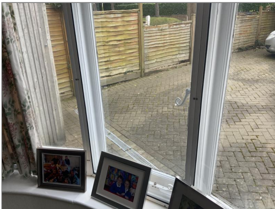
Photo - 33 Secondary glazing
