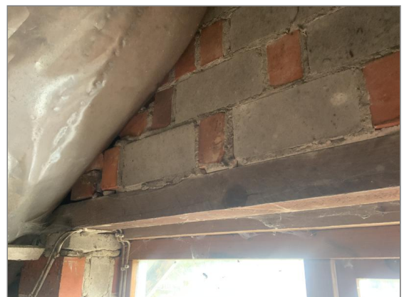
Photo - 26 Example of support to internal wall
