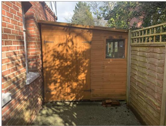
Photo - 77 Shed to side
