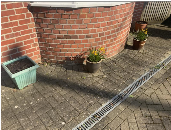
Photo - 23 Vent below
