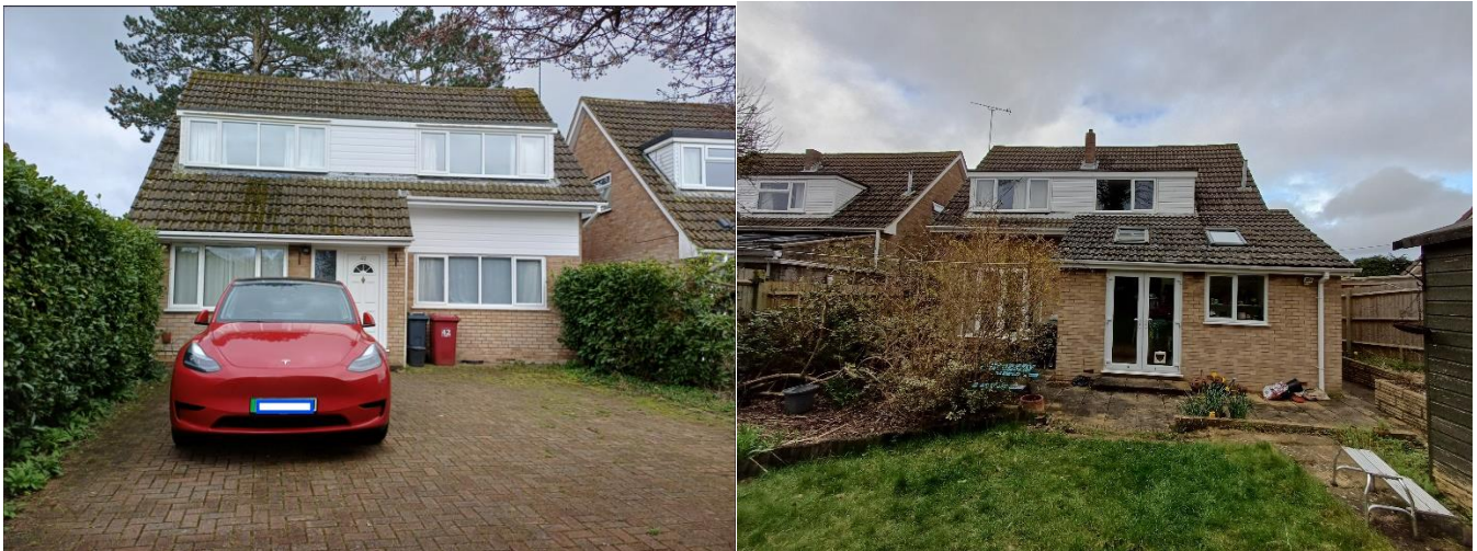
Figures 1 & 2: Front and rear views of 42 Silverthorne Drive, taken 27/02/2026
