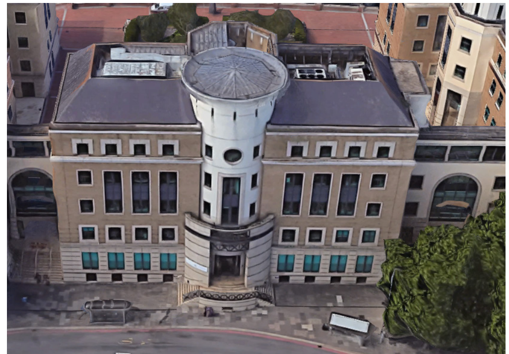
The Front (South) Elevation viewed from Kings Road
