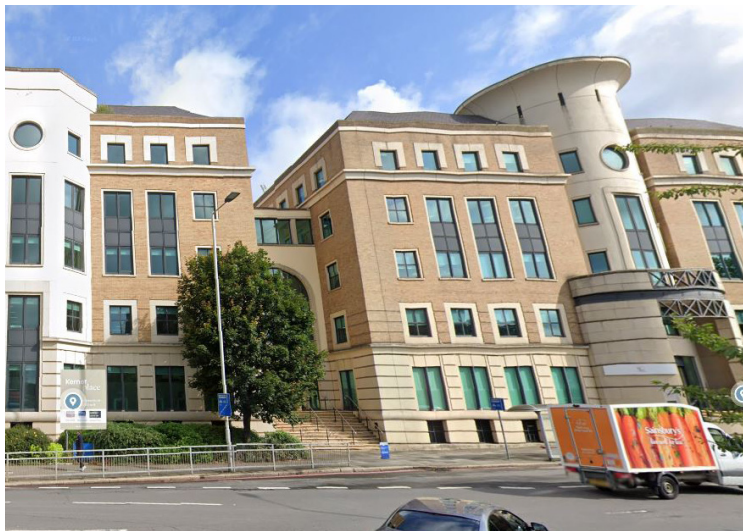
3 - South Elevation viewed from Kings Road
