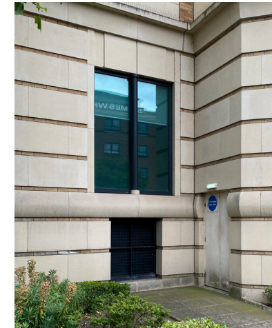
Example 2 - Existing ground floor raised fixed window in vicinity of fire escape door
