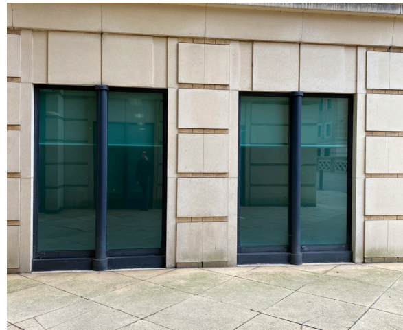
Example 1 - Typical existing ground floor fixed windows
