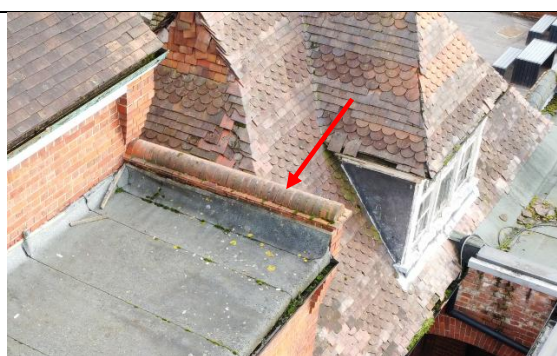
Fig 1.8 – Parapet to the edge of the southern flat roof
