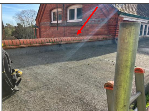
Fig 1.7 – Parapet to the edge of the northern flat roof
