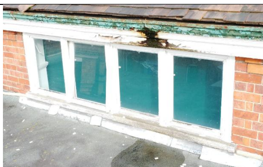
Fig 1.5 - Existing Windows above flat roofs
