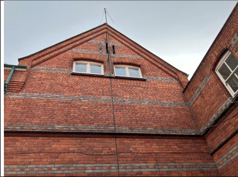
Photograph 10 English Block Northern Elevation
