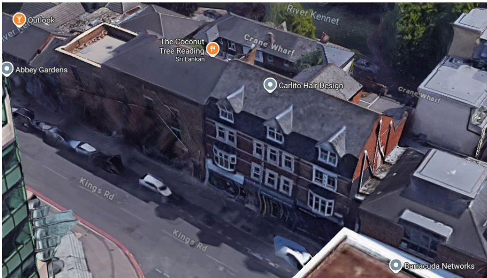
Fig.01 View of the site
