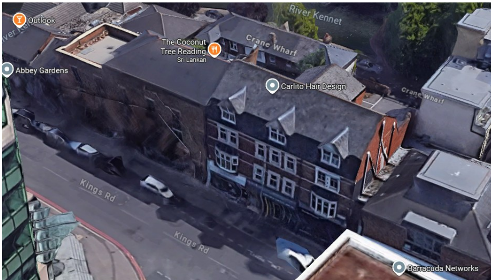
Fig.01 View of the site
