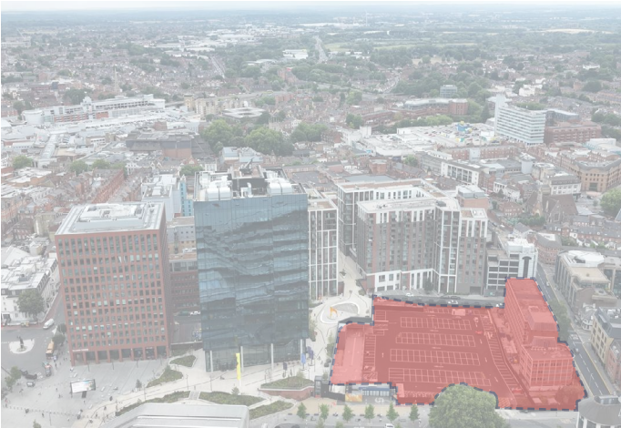
Station Hill existing site condition, looking south towards Friar Street
