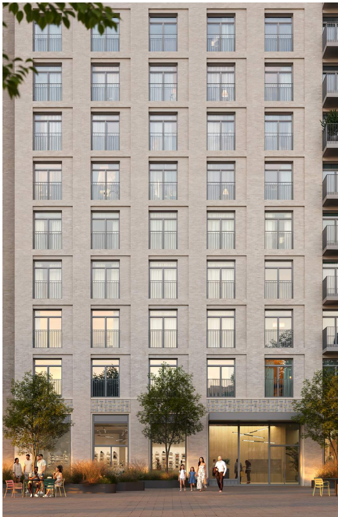
Enhanced facade detailing and material expression
