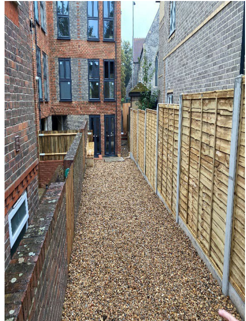
The existing fence was retained in line with drawing 202 P 09 Rev B.
