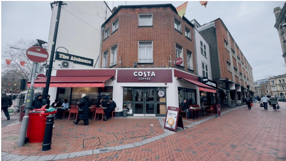
Plate 4 - Modern commercial shopfront and signage at Costa adjoining application site
