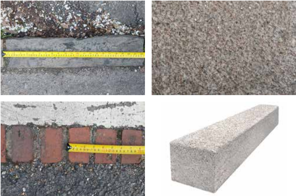
Top left: Existing granite highway kerbs Top right: New ‘Figueiredo’ Portuguese granite Bottom Left: Existing brick edgings Bottom Right: New Brecon ‘Black Fleck’ Conservation kerb
