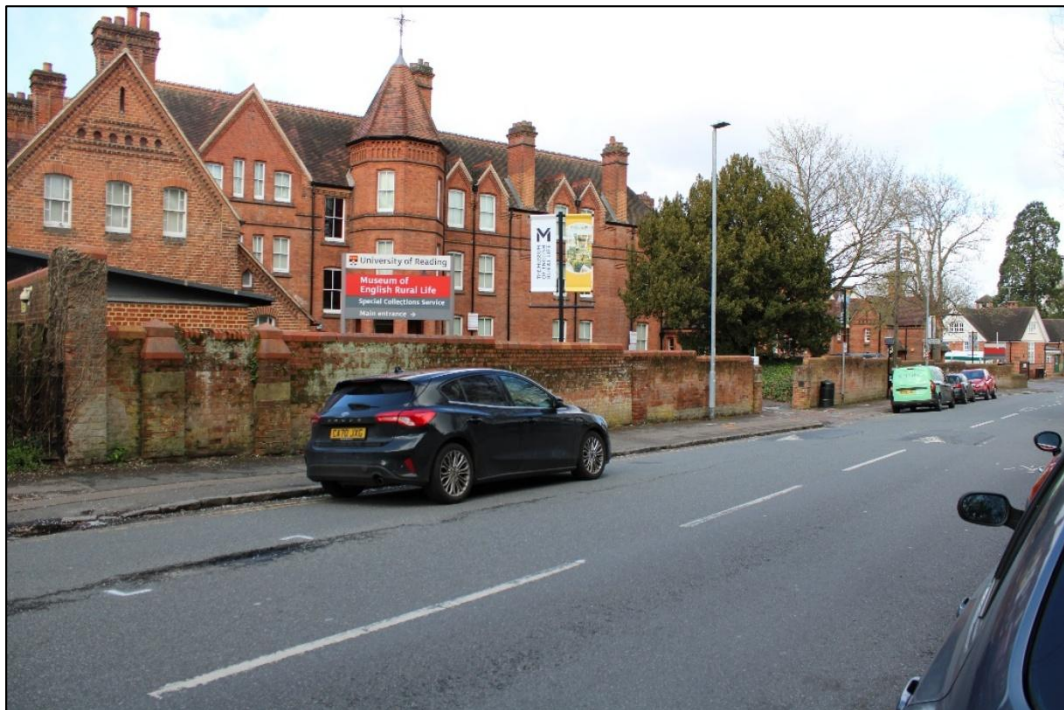
Figure 12. View towards the MERL from the southeast
