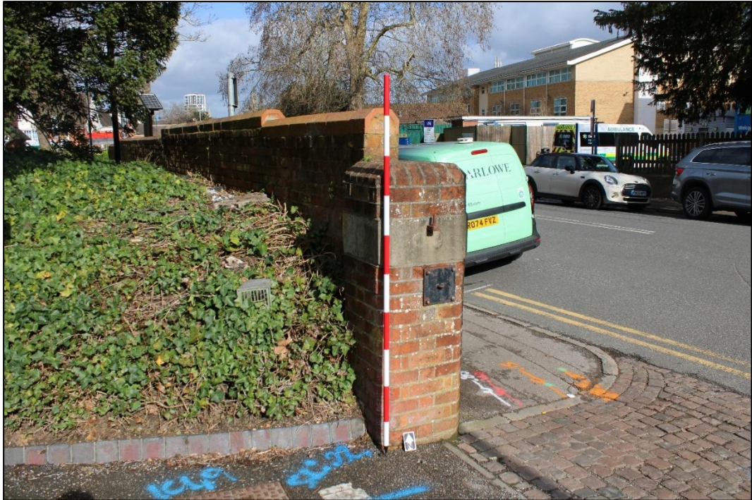
Figure 20. View of existing southern entrance / exit onto Redlands Road from MERL brick pier looking northeast
