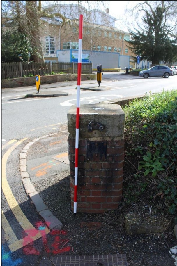
Figure 30. View of the vehicular access to / from Acacia Road junction of MERL east brick pier looking southeast
