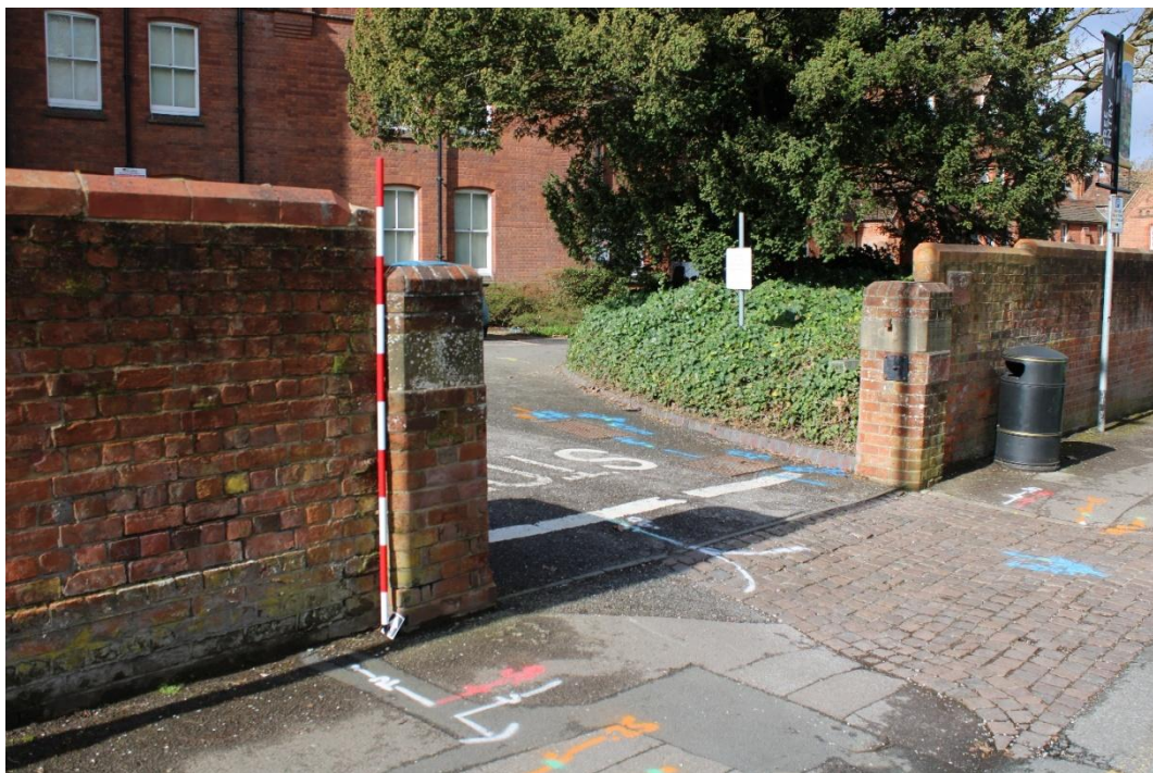
Figure 15. View of extant existing southern entrance / exit onto Redlands Road from MERL brick piers
