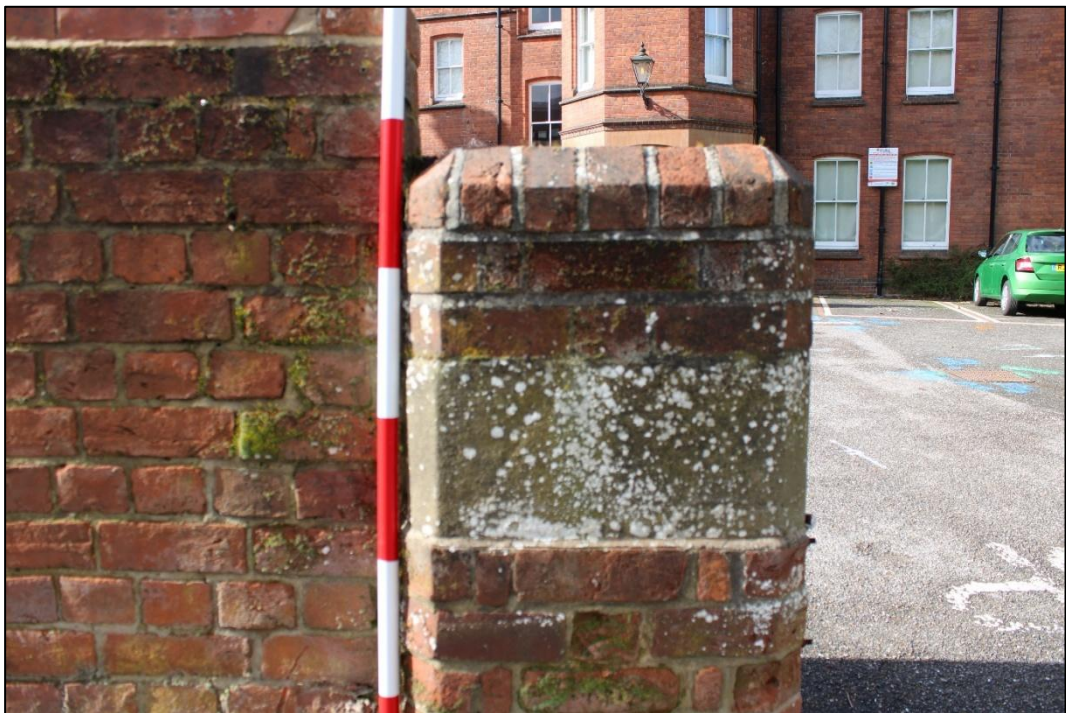
Figure 17. Sample view of stone cap on south pier of the existing southern entrance / exit onto Redlands Road from MERL
