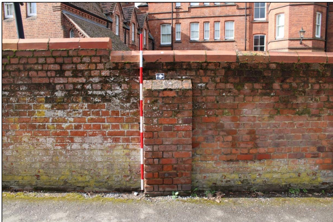
Figure 25. Sample view of red brick wall buttress
