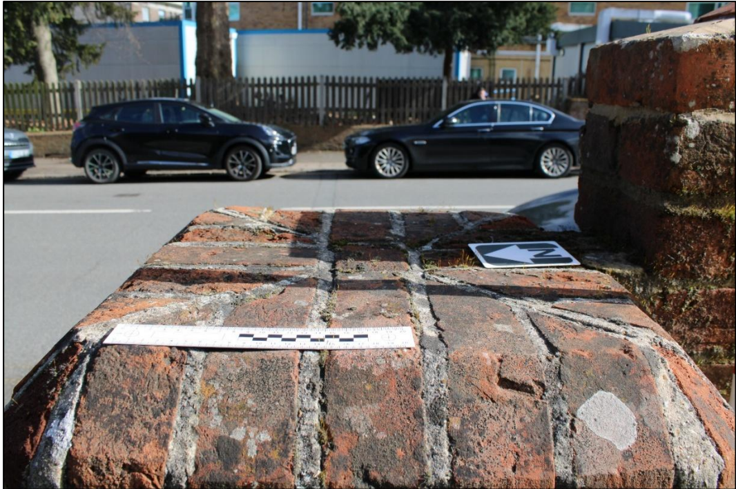
Figure 22. Sample view of brick pier cap
