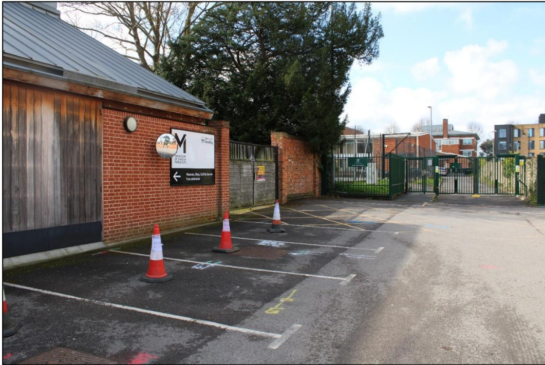
Figure 13. View of red brick boundary wall along Acacia Road
