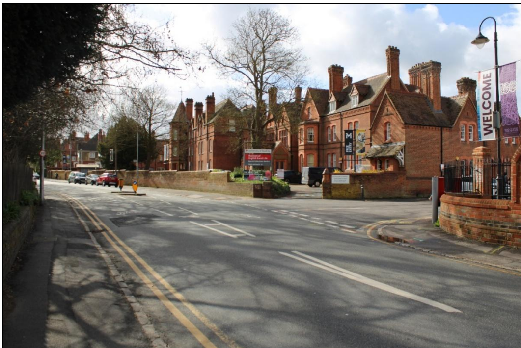
Figure 11. View towards the MERL from the northeast
