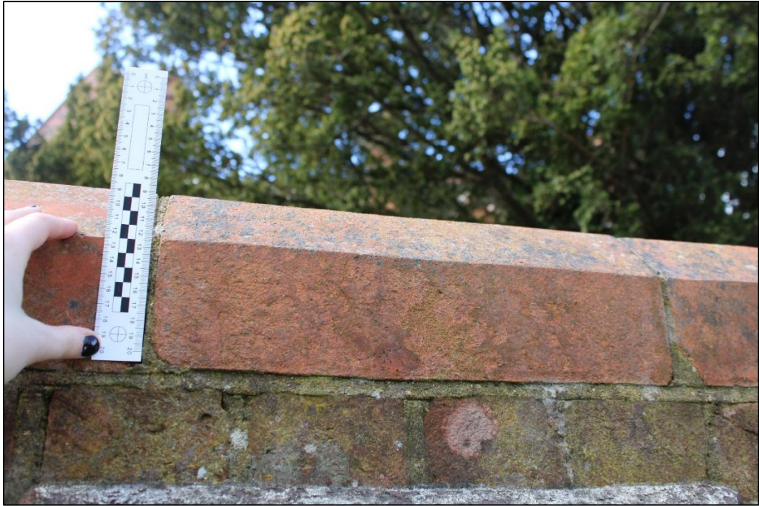
Figure 34. Sample view of sandstone coping
