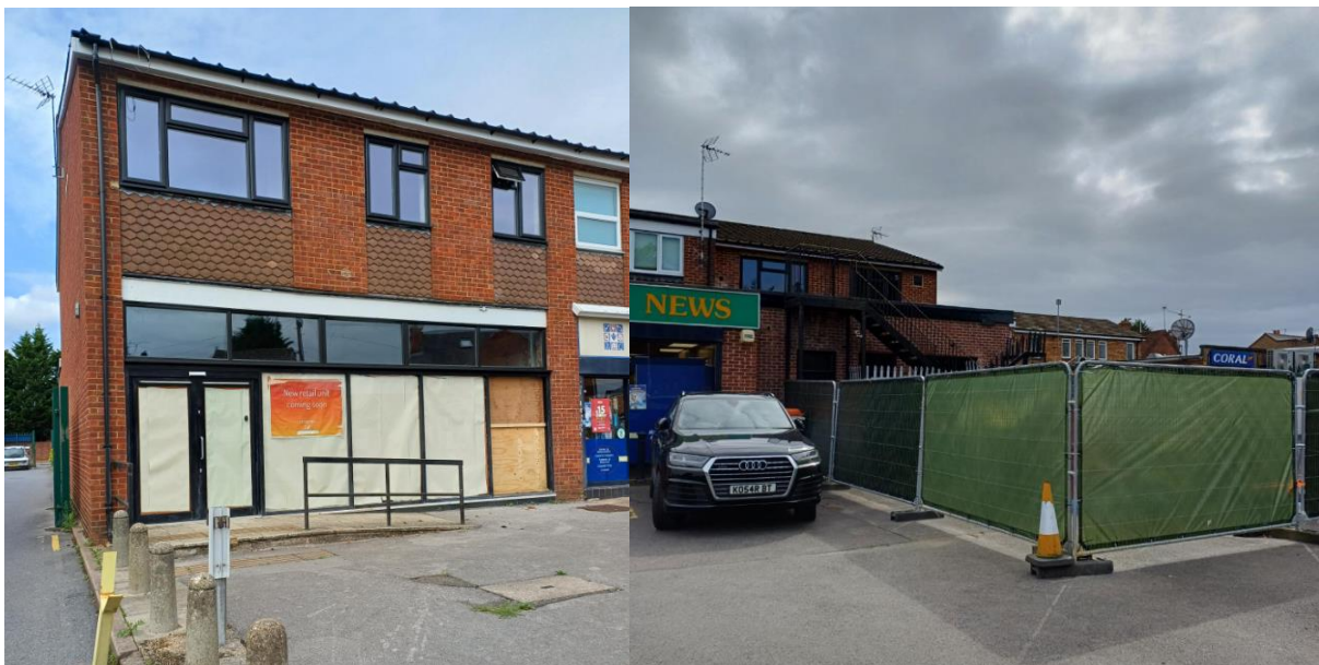
Left: Application site as seen from School Road. Right: Rear of the site. Images taken by planning officer on 09/09/24.
