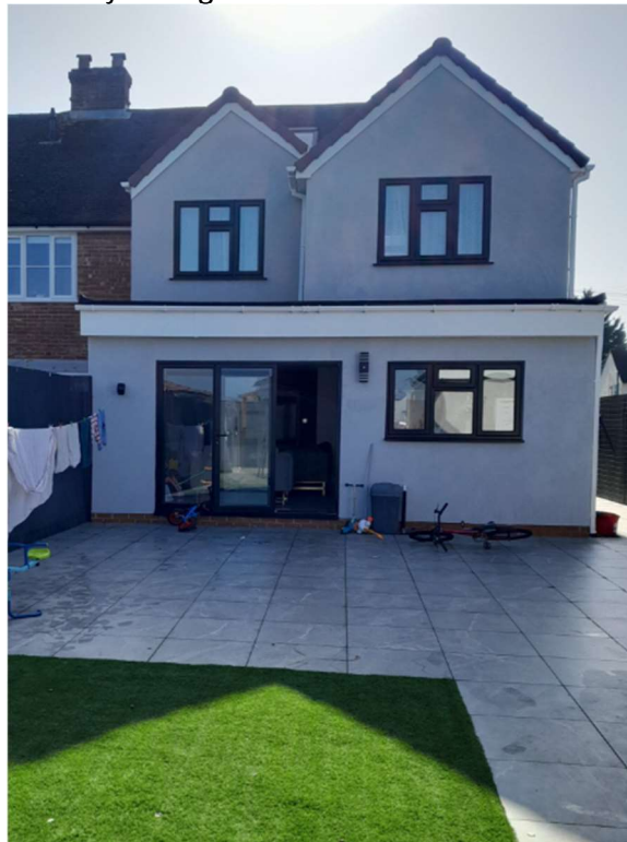
Looking south towards northerly elevation of 193 Hartland Road.
