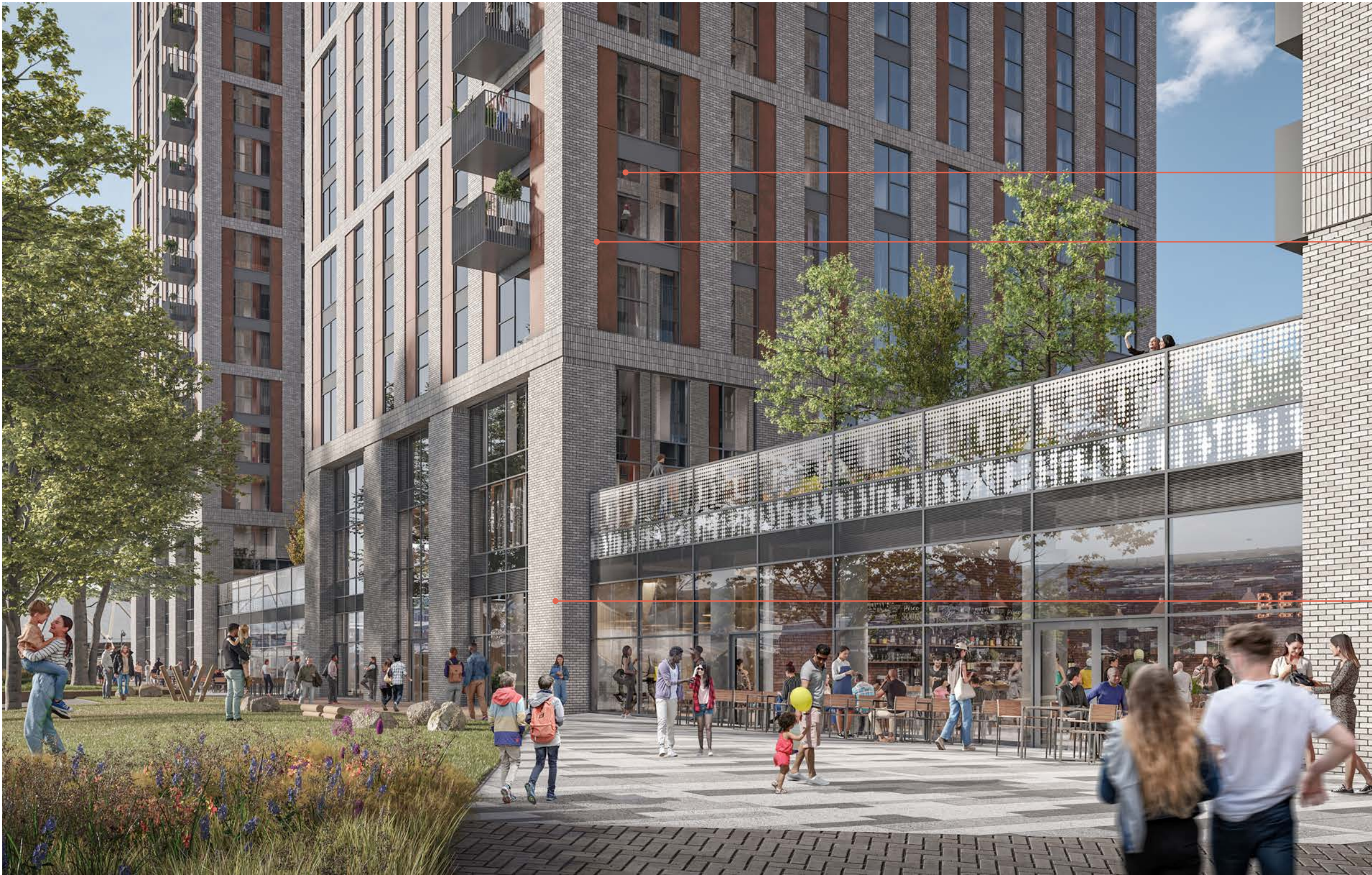
The residential building bases are given a grand 3 storey language contrasting with the lightweight glazed façades in between..
