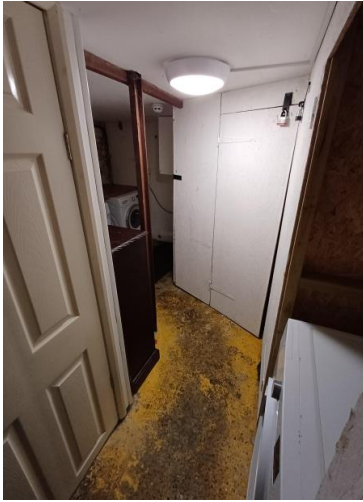
Utility room and bathroom door at basement floor level
