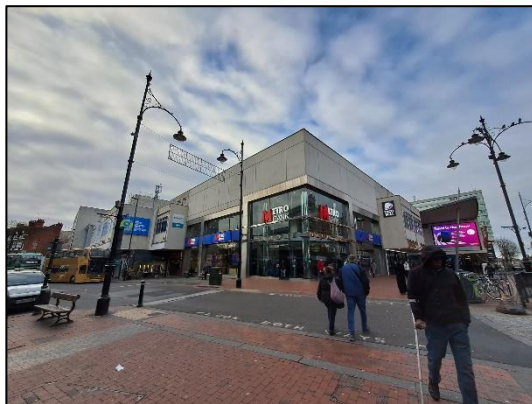
Photo 1. North-east elevation of Broad Street Mall with Fountain House above.
