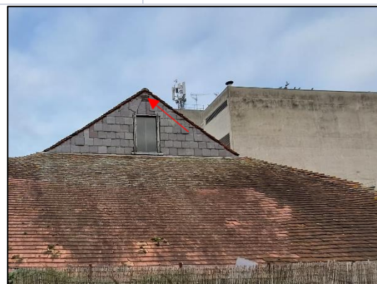
Photo 10. View of potential roost features present on Building 2.
