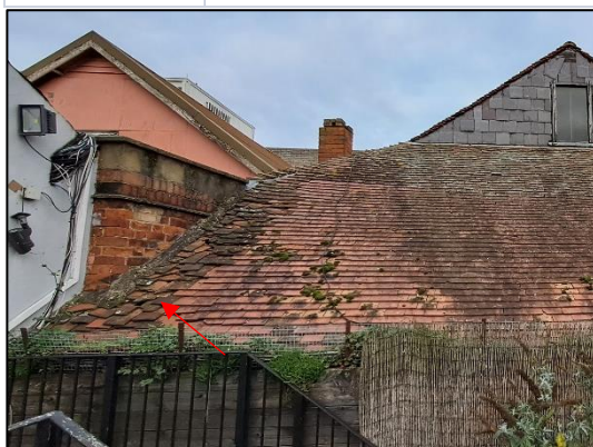
Photo 9. View of potential roost features present on Building 1.
