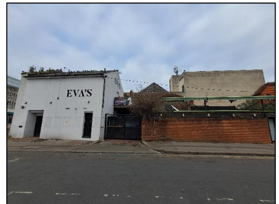
Photo 4. South elevation of Eva's building and barn house.
