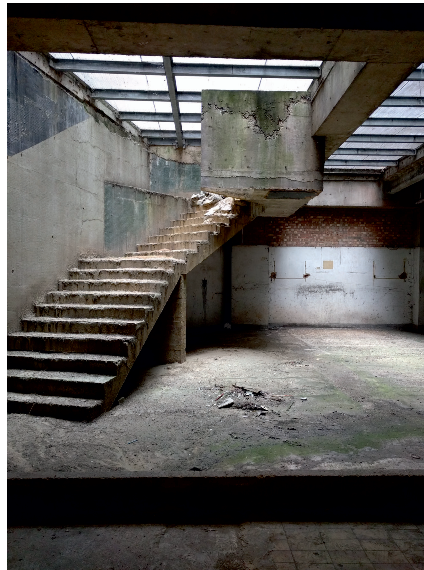
Fig 12 North-west facing view of basement at Broad Street Mall (MOLA photograph, 28/06/2018)
