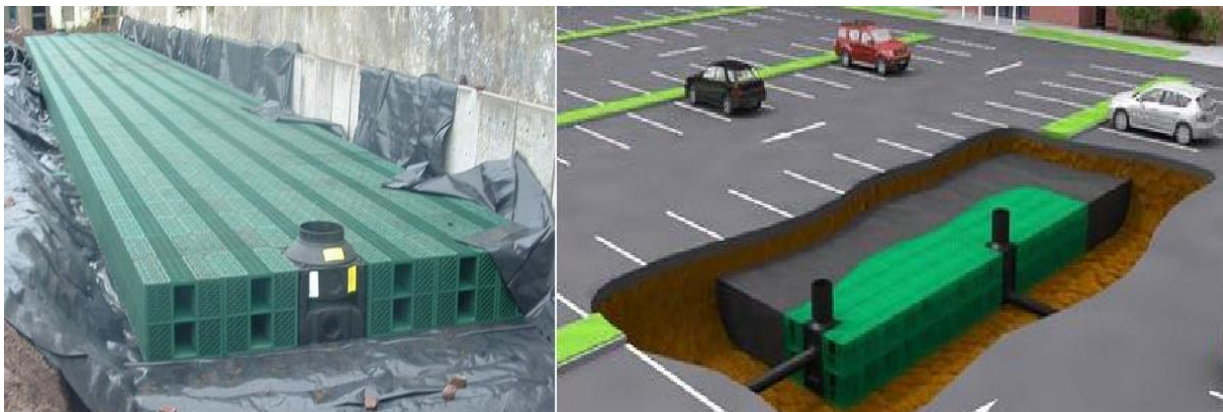
Figure 12: Typical cellular attenuation tank
