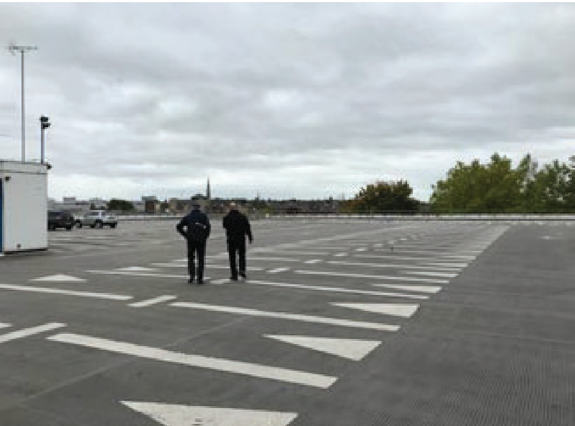
Figure 5 Second Storey Roof Car Park, above the Broad Street Mall Shopping Centre
