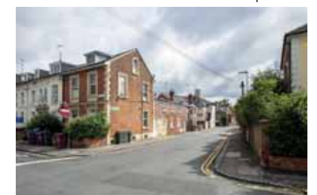
22 Junction with Baker Street and Jesse Terrace
