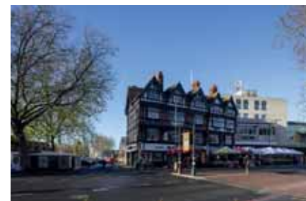
7 From in front of Reading Minster looking west directly towards 21-23 St Mary's Butts
