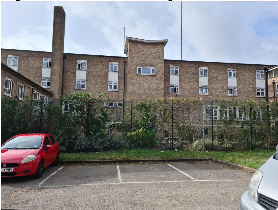
Image 2 – View to Existing Rear Elevation to West
