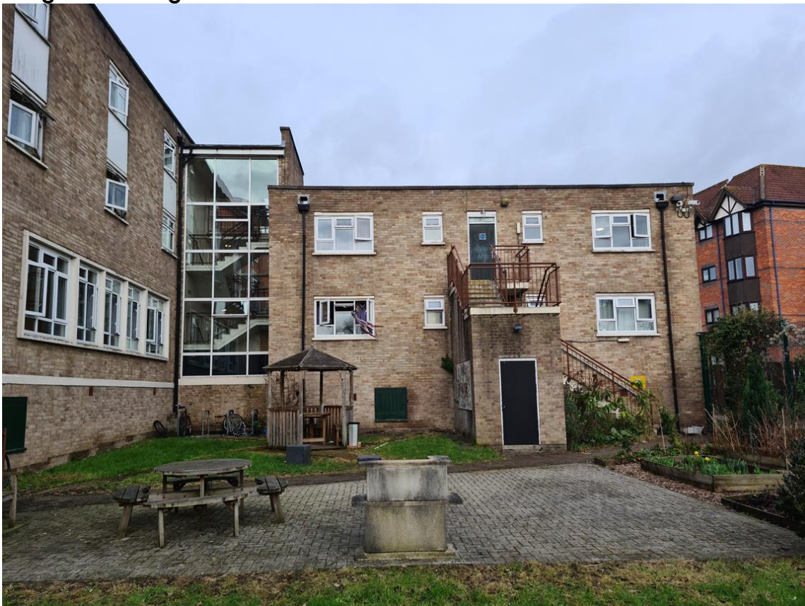
Image 4 – Existing Rear Garden Area to North West
