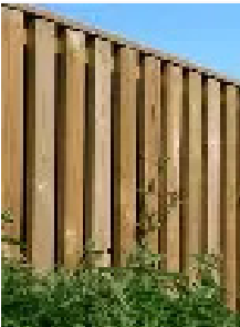
Plant & Refuse Enclosures
