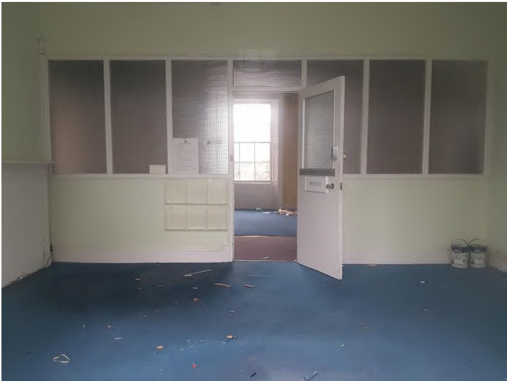
Plate 4: View south showing some of the rooms inside Yeomanry House.
