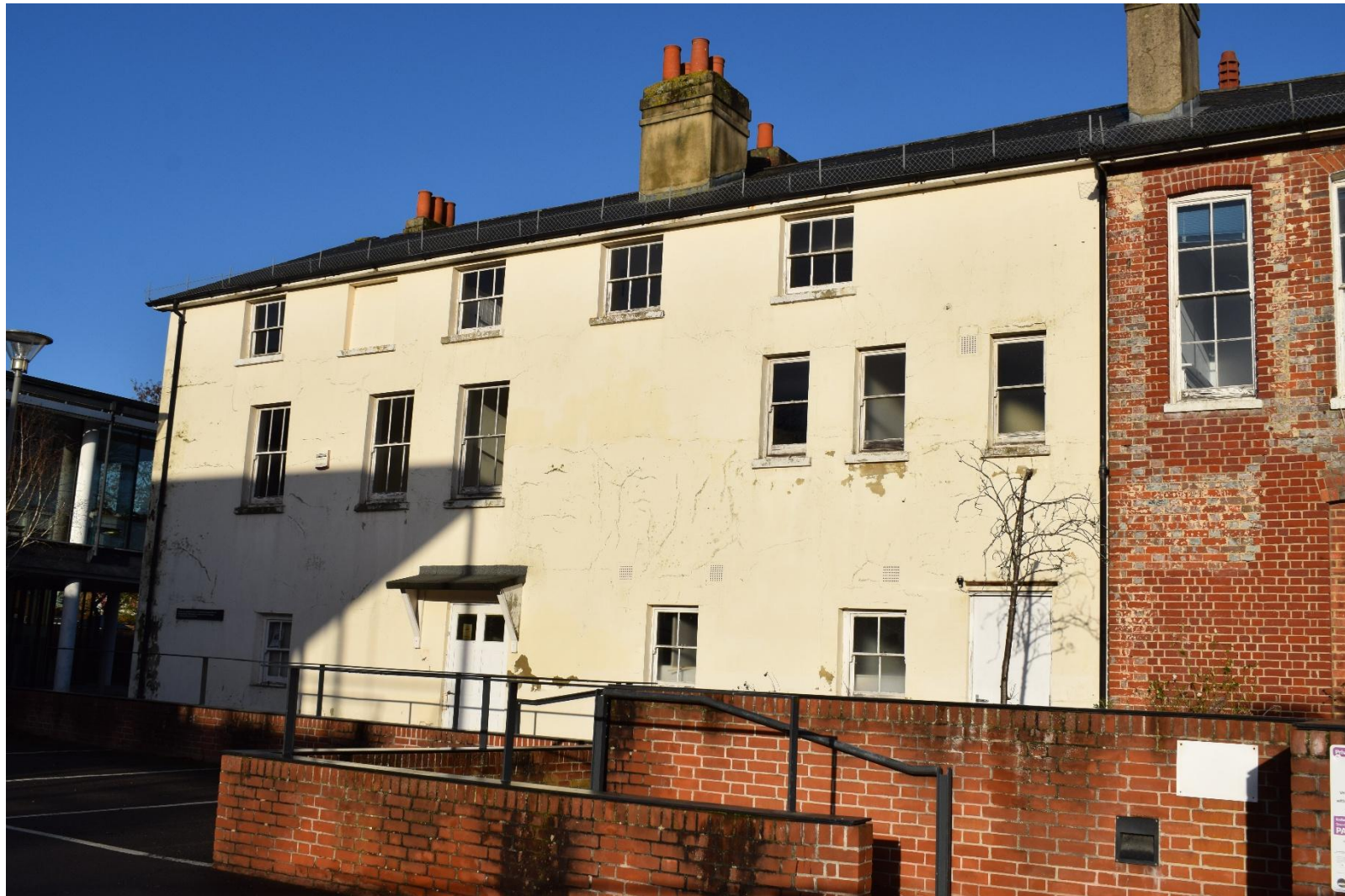
Figure 11: The rear elevation of Phases 2a and 2b
