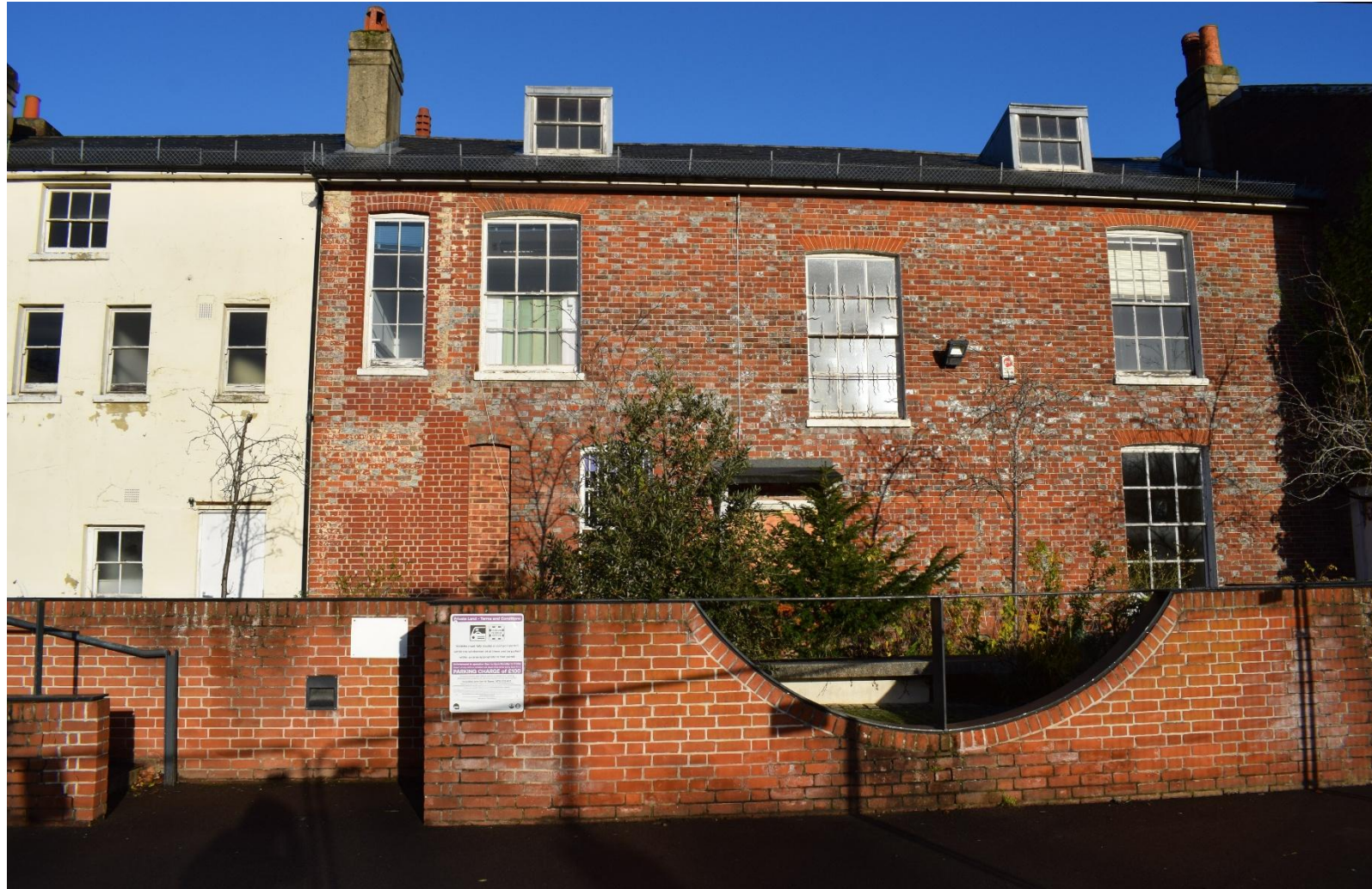
Figure 9: The rear elevation of Phase 1, the original core of Yeomanry House
