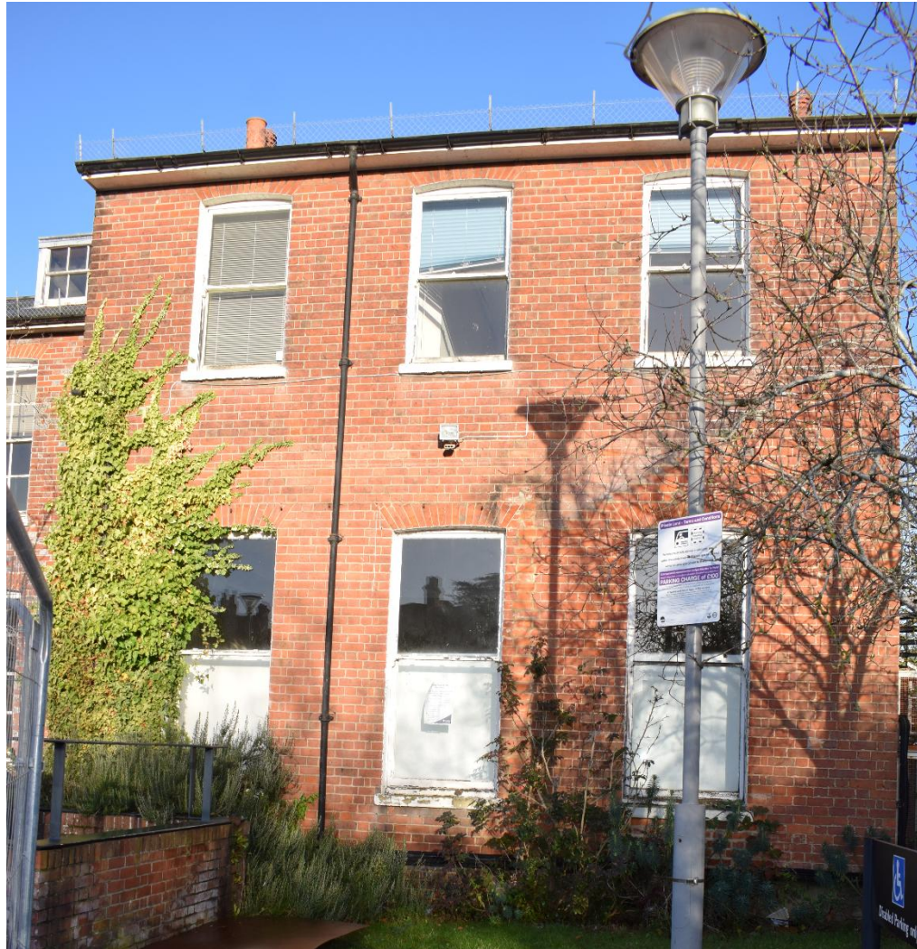
Figure 14: The rear elevation of Phase 3
