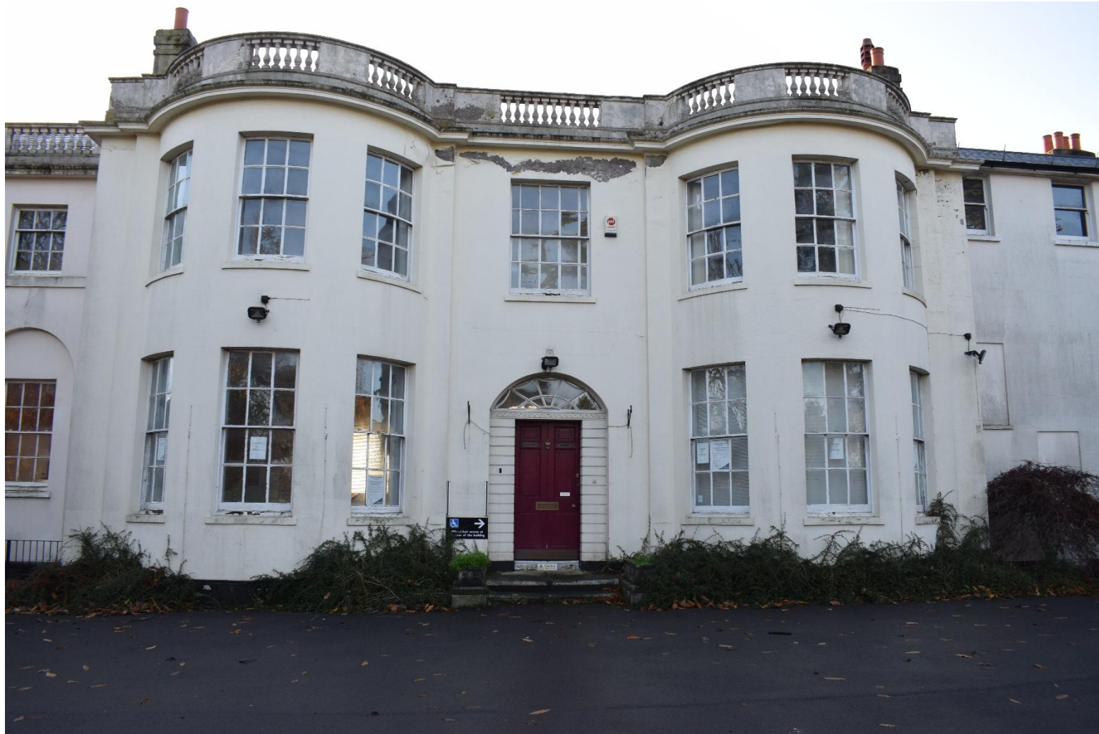
Figure 7: The frontage of Phase 1, the original core of Yeomanry House
