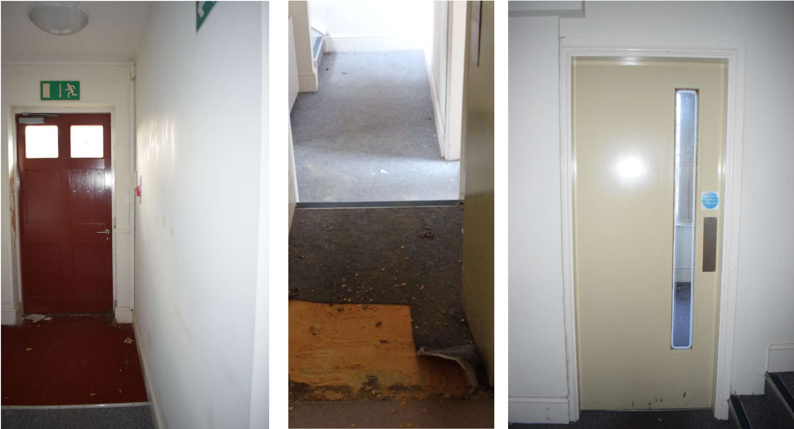
Plate 64 Reconfigured spaces: This image illustrates one of the reconfigured spaces, and associated fire door exits. Inset: a detail of the solid flooring on the ground floor of Phase 2, due to re-modernisation.
