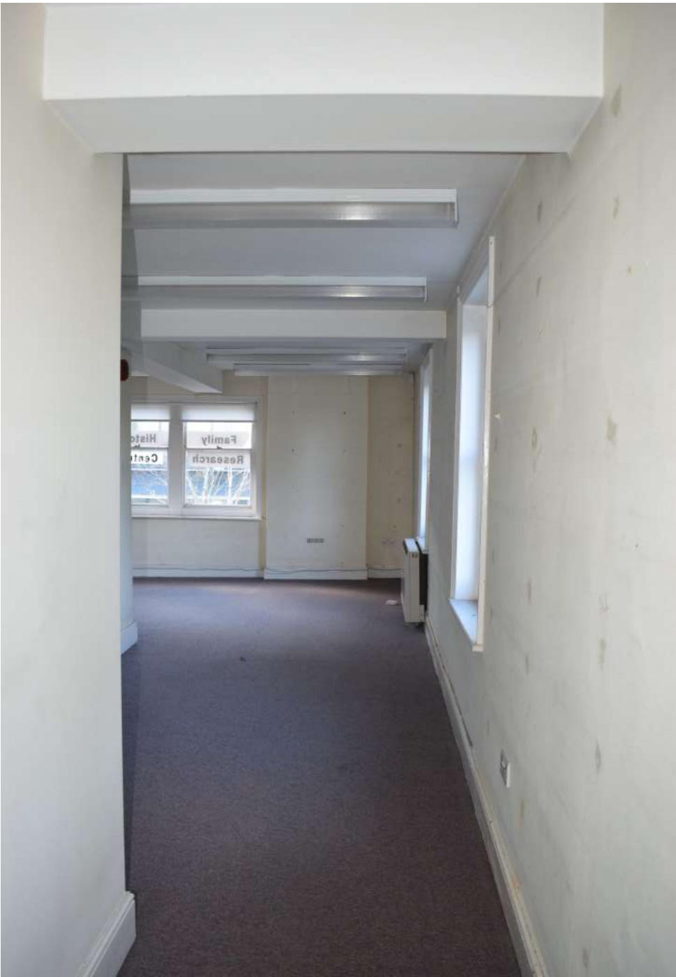
Plate 70 Reconfigured spaces: This image displays the reconfigured first-floor Exhibition Room, showing a series of downstands spanning the space created for the enlarged room.
