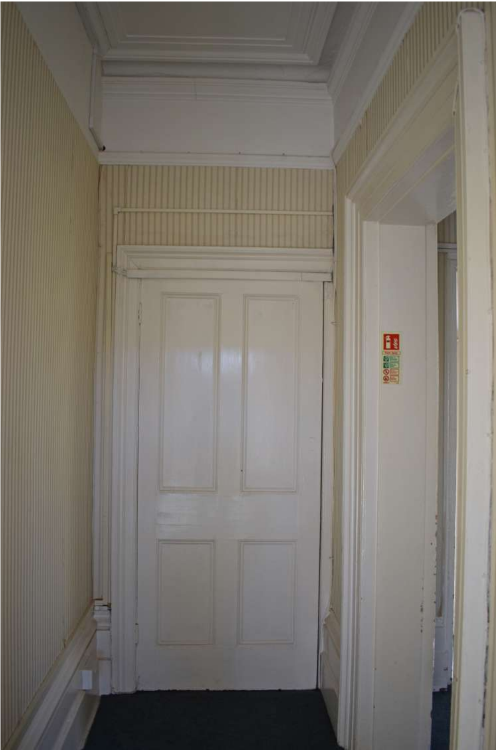
Plate 120 The skirtings in the eastern corridor are high and highly decorative, and there is a picture rail indicating a sub-division of a significant room, now Offices A and B and the kitchenette.
