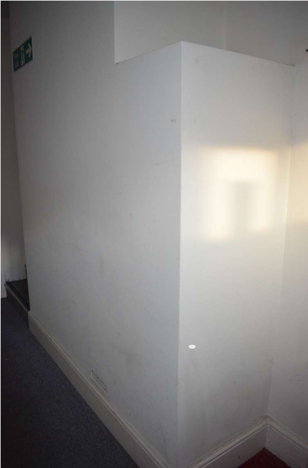
Room 19a - Historic fire place in the corridor by the fire exit
