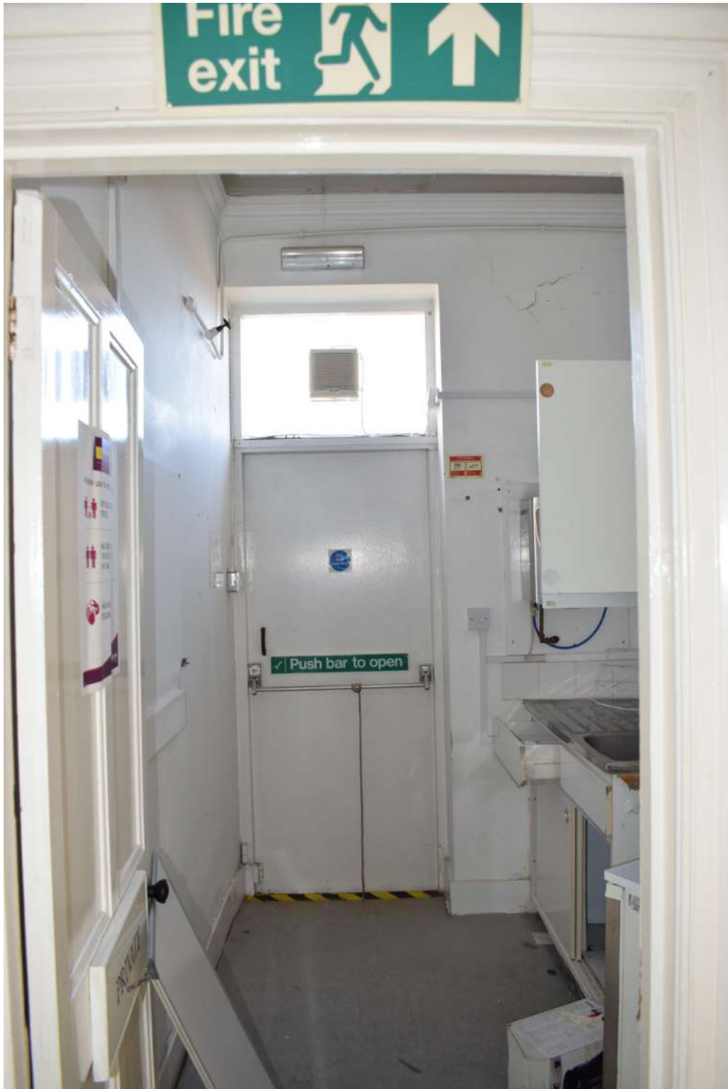
Plate 128 The doorway to the kitchenette appears to be a modern insertion. Inset: a detail of the timber flooring.
