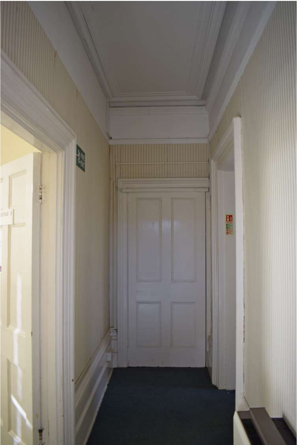
Plate 120 The skirtings in the eastern corridor are high and highly decorative, and there is a picture rail indicating a sub-division of a significant room, now Offices A and B and the kitchenette.
