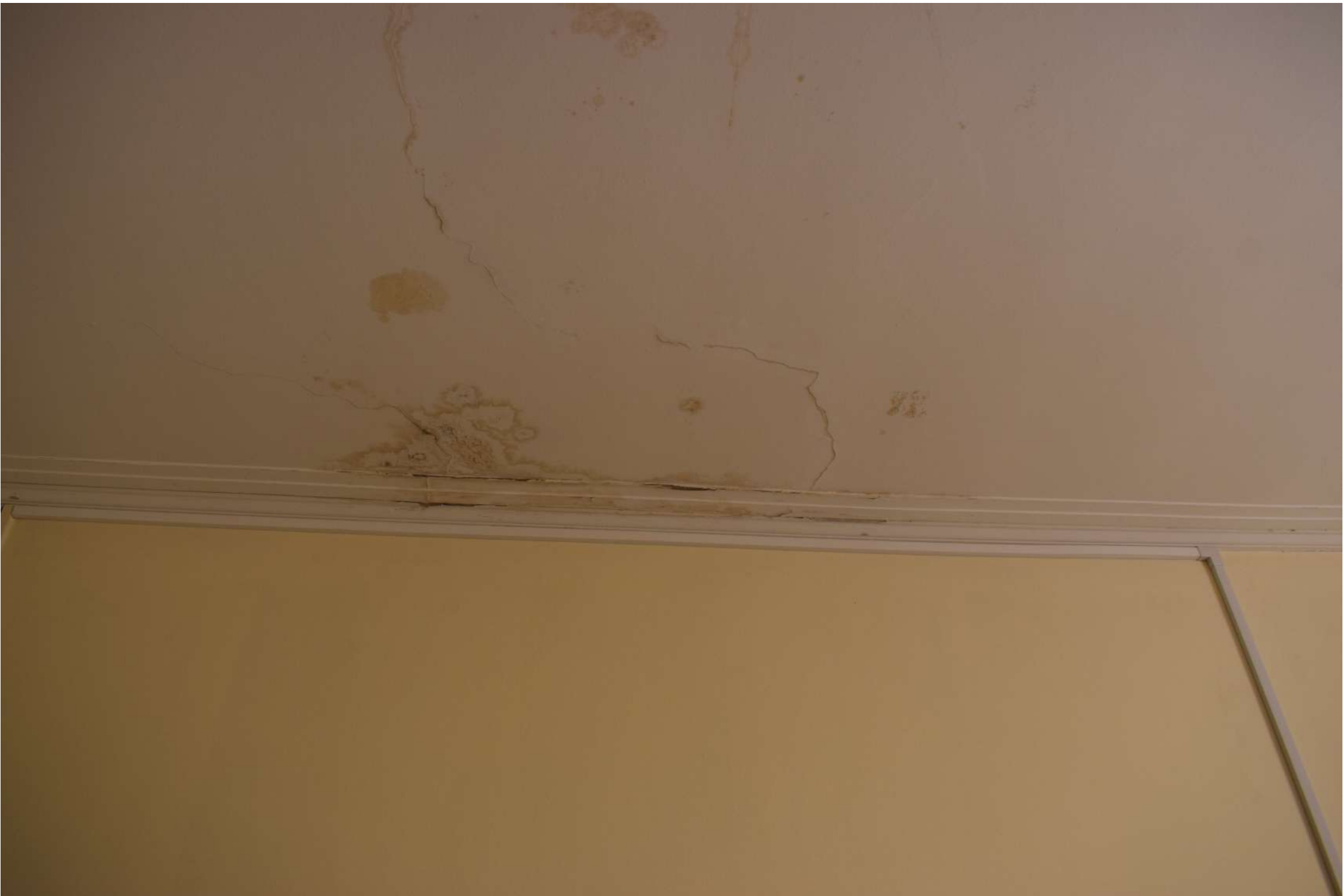
Plate 123 In Office B, a damp stain caused by water ingress into the ceiling, affecting what appears to be a modern and historic coving. Inset: a detail of the timber flooring.
