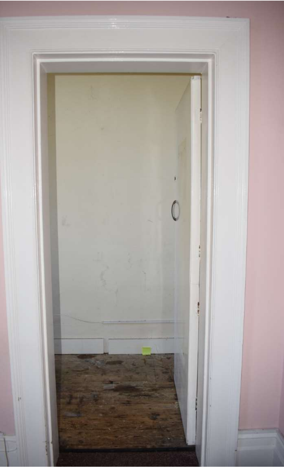
Plate 108 This angled wall that cuts into window architrave. The angled wall cutting into the window architrave is often seen when an original room layout (like a hallway or main reception room) was subdivided later to create a smaller, functional space, such as a butler's pantry or washroom. Insets: a detail of a poorly executed repair that took part of the lath and plaster ceiling with it and the timber flooring.
