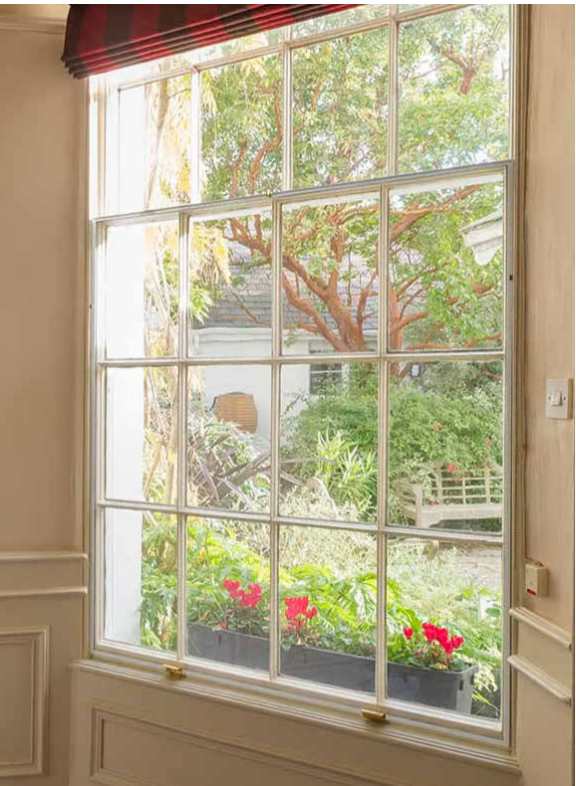
Type 3 - secondary glazing to individual sashes (mitchellanddickinson.co.uk)
