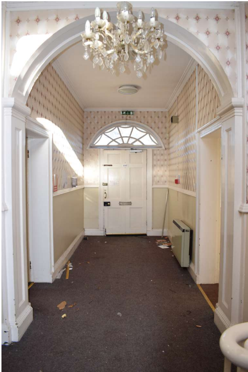
Plate 1 General photographs of the entrance hallway illustrating the presence of non-decorative coving, relatively decorative, low-profile skirting, and a historically retained dado rail.
