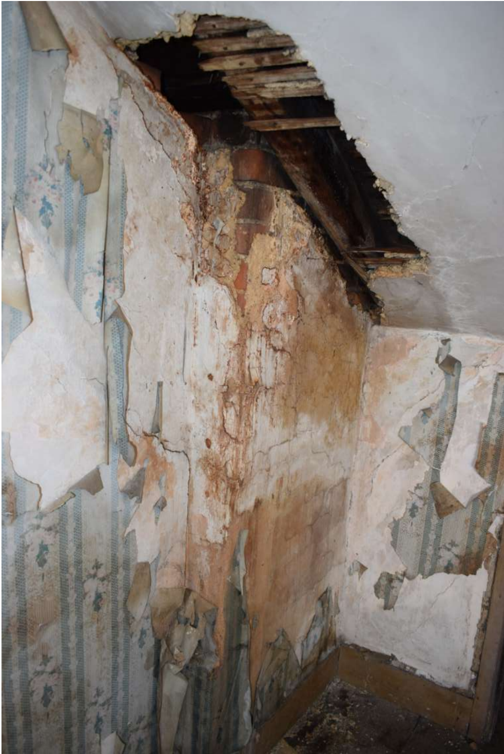
Attic Room 18 - Eastern storeroom
