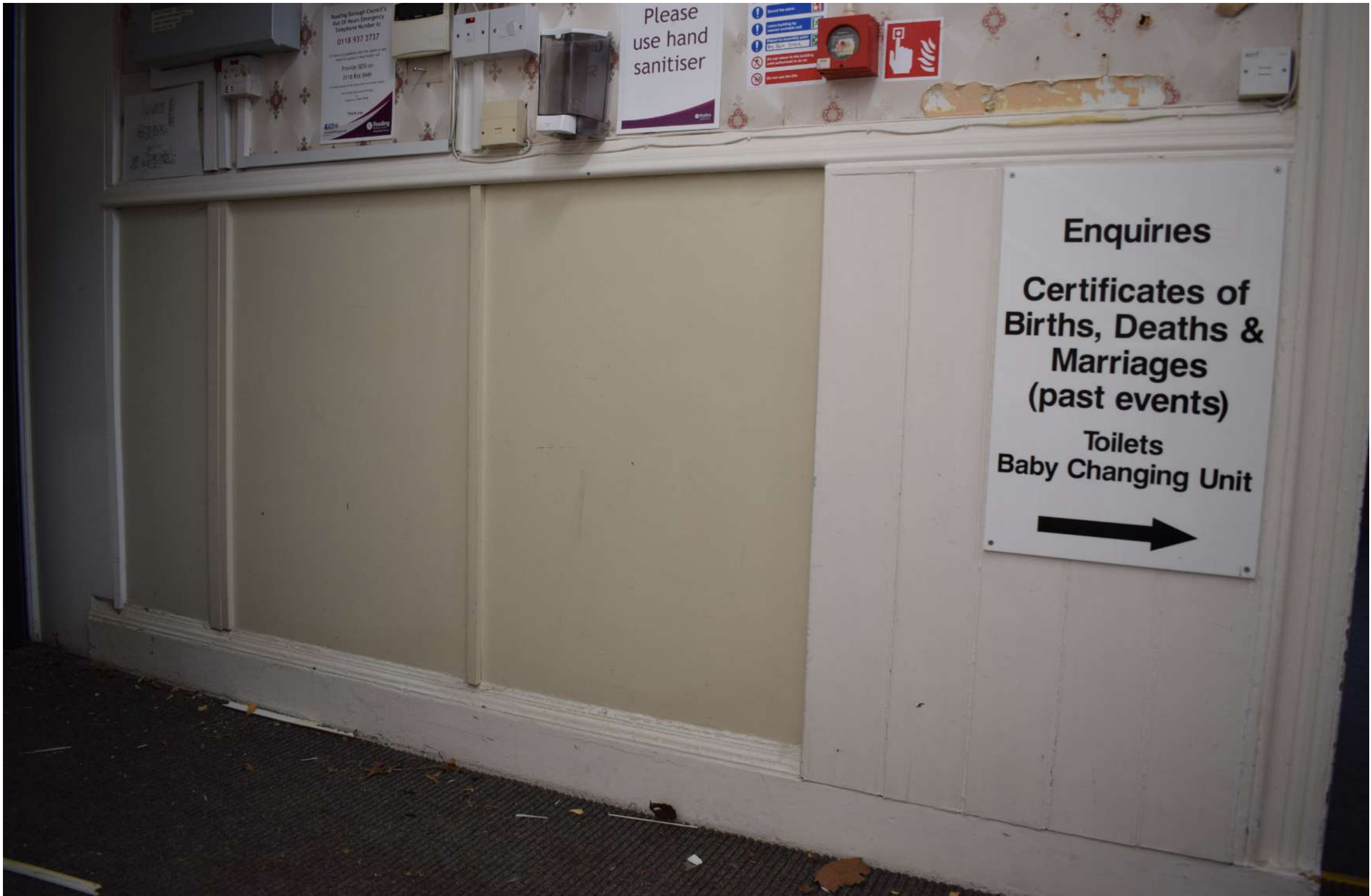
Plate 3 Detailed image confirming the apparent absence of wall panelling below the existing dado rail height.
