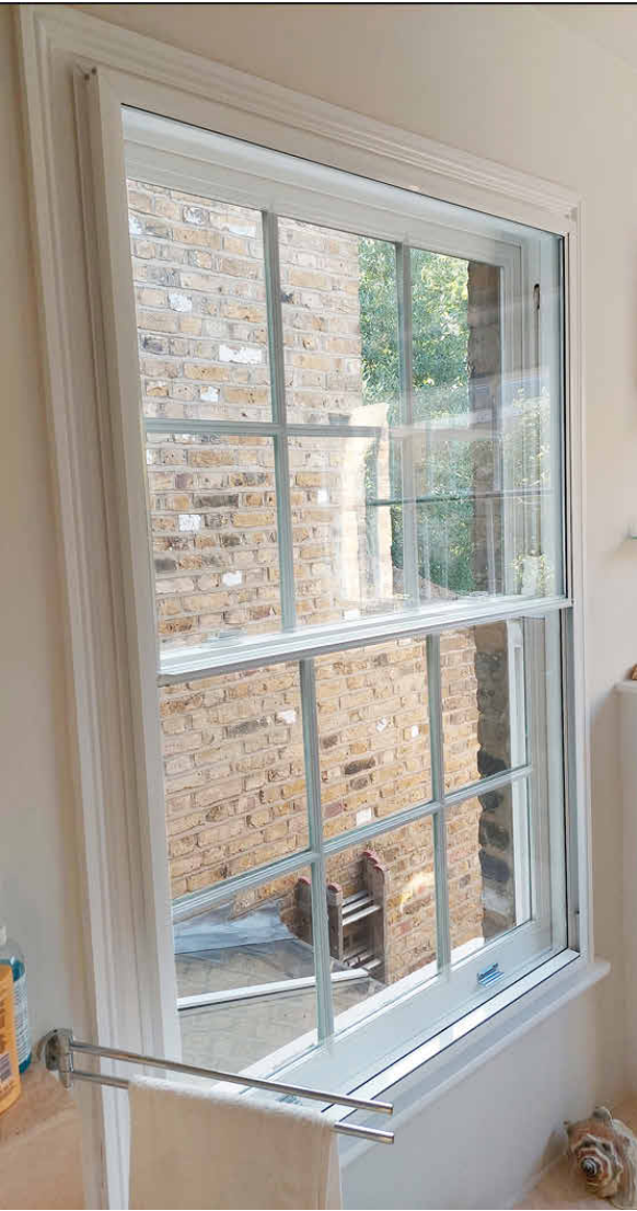
Type 4 - Entire window covered with mechanically fixed toughened glass secondary glazing (northlondonglazing.com)
