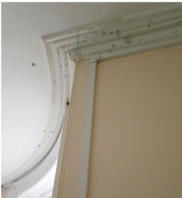
Plate 1: The photos above show the area of lead theft on the roof and those below the damage to second floor ceiling and floor. Where lath and plaster has been replaced, and joists repaired, these have been exposed due to the damage.
