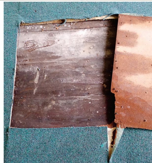
Plate 1: The photos above show the area of lead theft on the roof and those below the damage to second floor ceiling and floor. Where lath and plaster has been replaced, and joists repaired, these have been exposed due to the damage.
