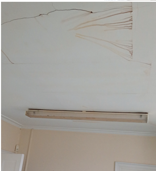
Plate 1: The photos above show the area of lead theft on the roof and those below the damage to second floor ceiling and floor. Where lath and plaster has been replaced, and joists repaired, these have been exposed due to the damage.
