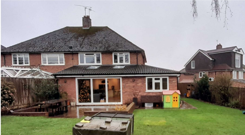
Existing rear elevation and context around property.
