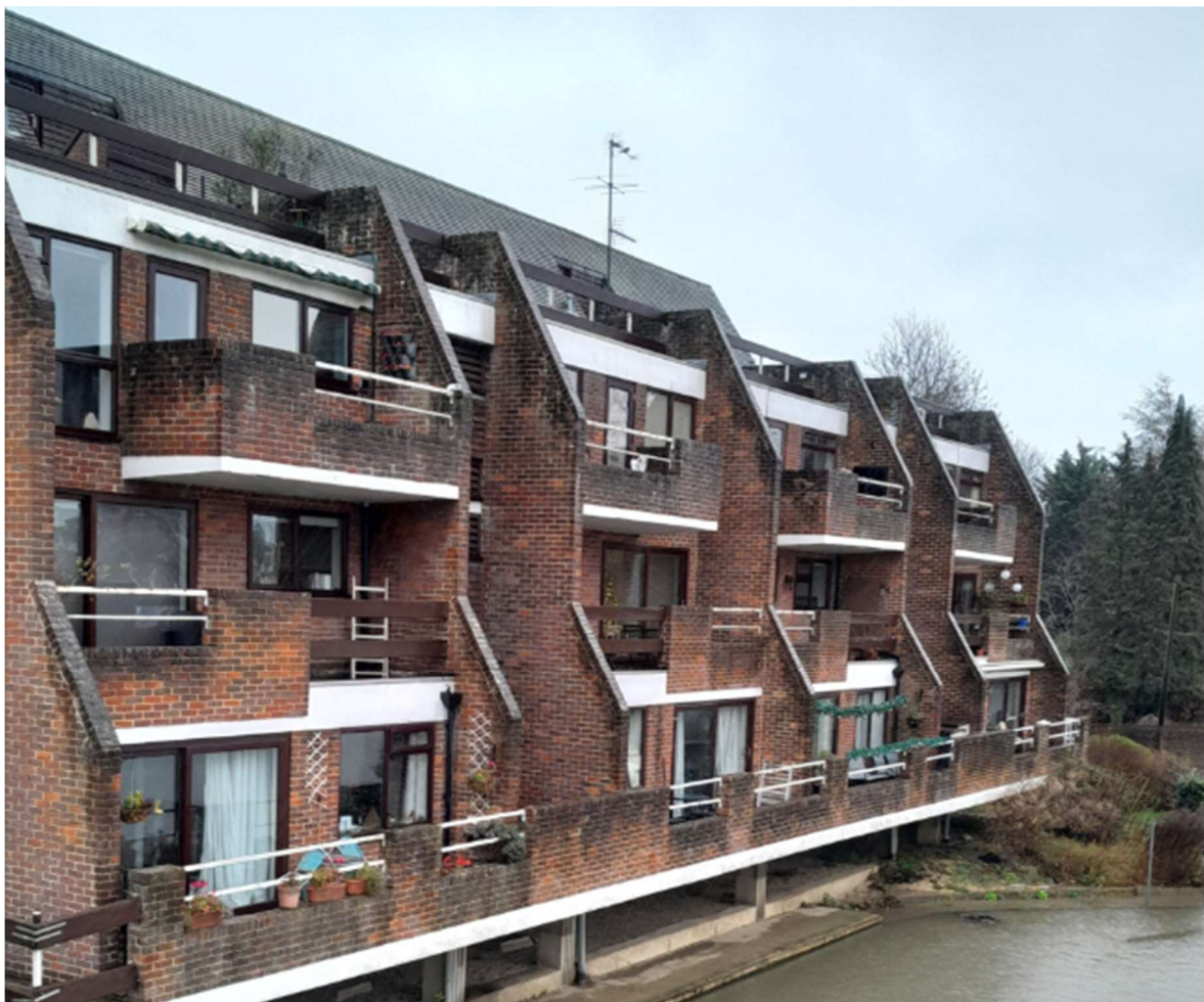
Block 2 – southwest facing elevation.
