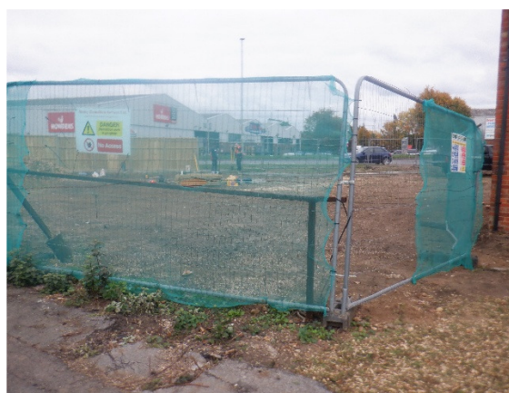
Photograph 2. The recently cleared site viewed from the south east.
