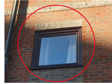
South Elevation Single window
