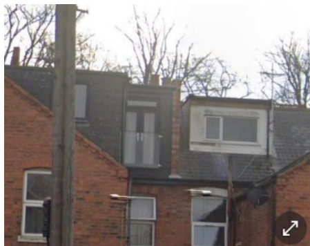
Rear prior to works
