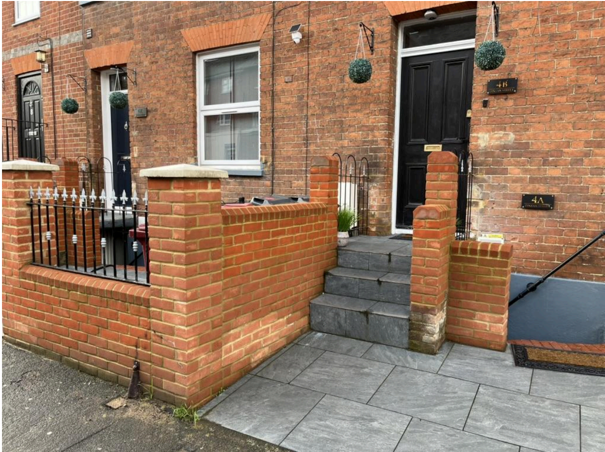
Recent Example of Boundary Wall 6, 4 Zinzan Street
