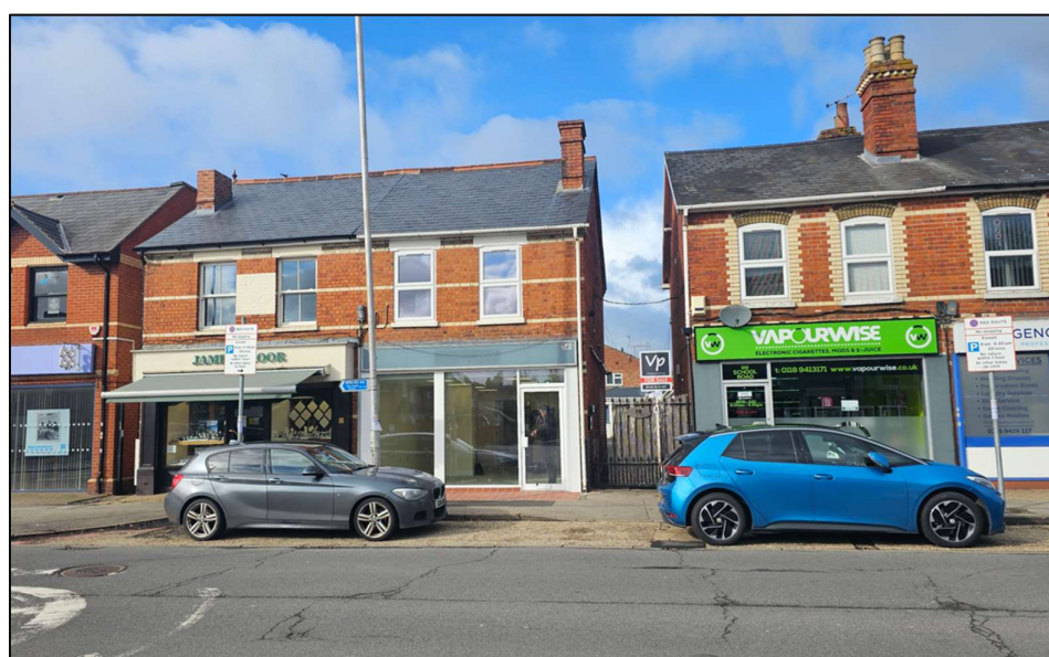
Figure 3: Photograph showing front elevation of existing building
