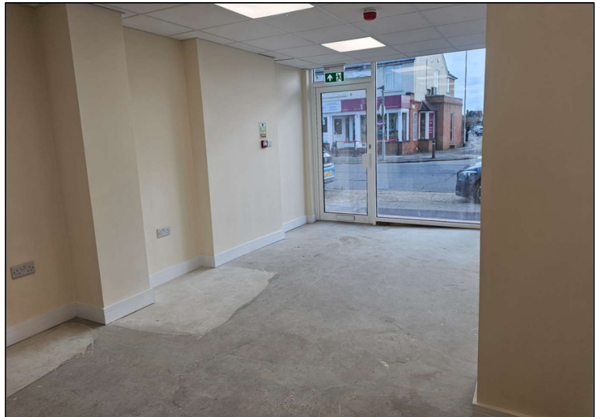
Figure 5: Photograph of interior view
