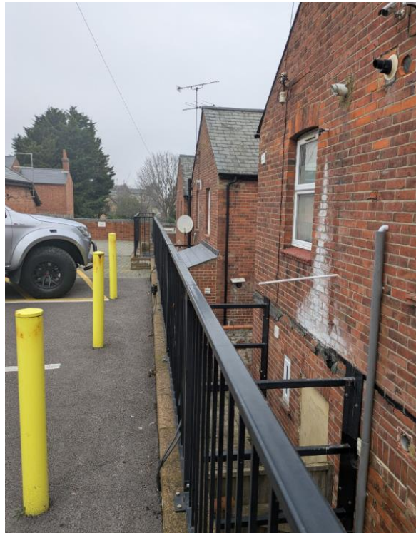
Image taken by case officer on site in 2025 showing the rear elevations of the properties on Southampton Street, the application site car park being on the left.
