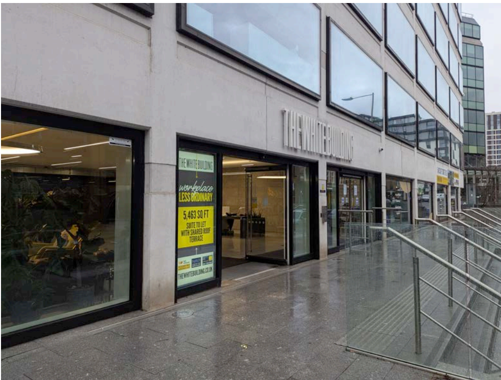
As Existing: Detail - Jan 2026
