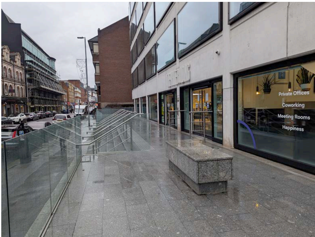
As Existing: Detail - Jan 2026
