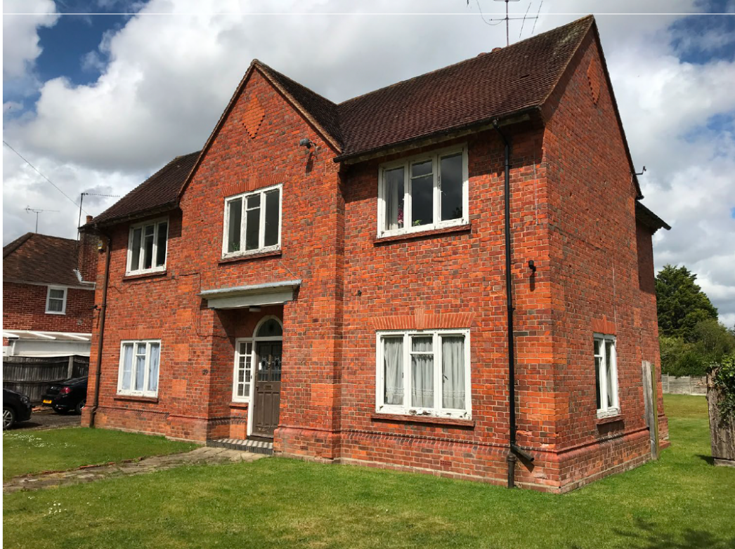
Figure 3: Appearance of the dwelling prior to application PL/21/1552 (used with permission of Hives Architects)
