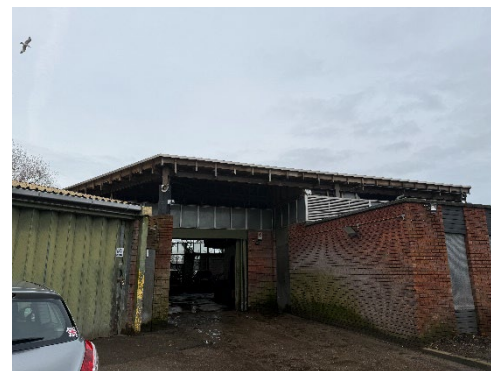
View of B1 facing west
