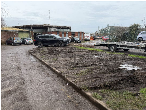
View facing west across the site
