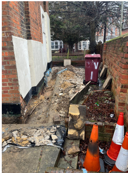
Plate 1 – a line of paving slabs lifted and sub-base removed alongside the building. T1 can be seen in the background.
