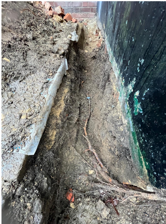
Plate 3 – Root bifurcates at the corner of the building and wraps around the corner of the building into the area proposed for the new steps
