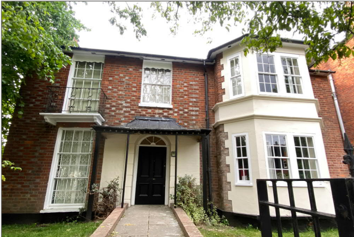
Image 16: View of the south elevation of Whitley Villa
