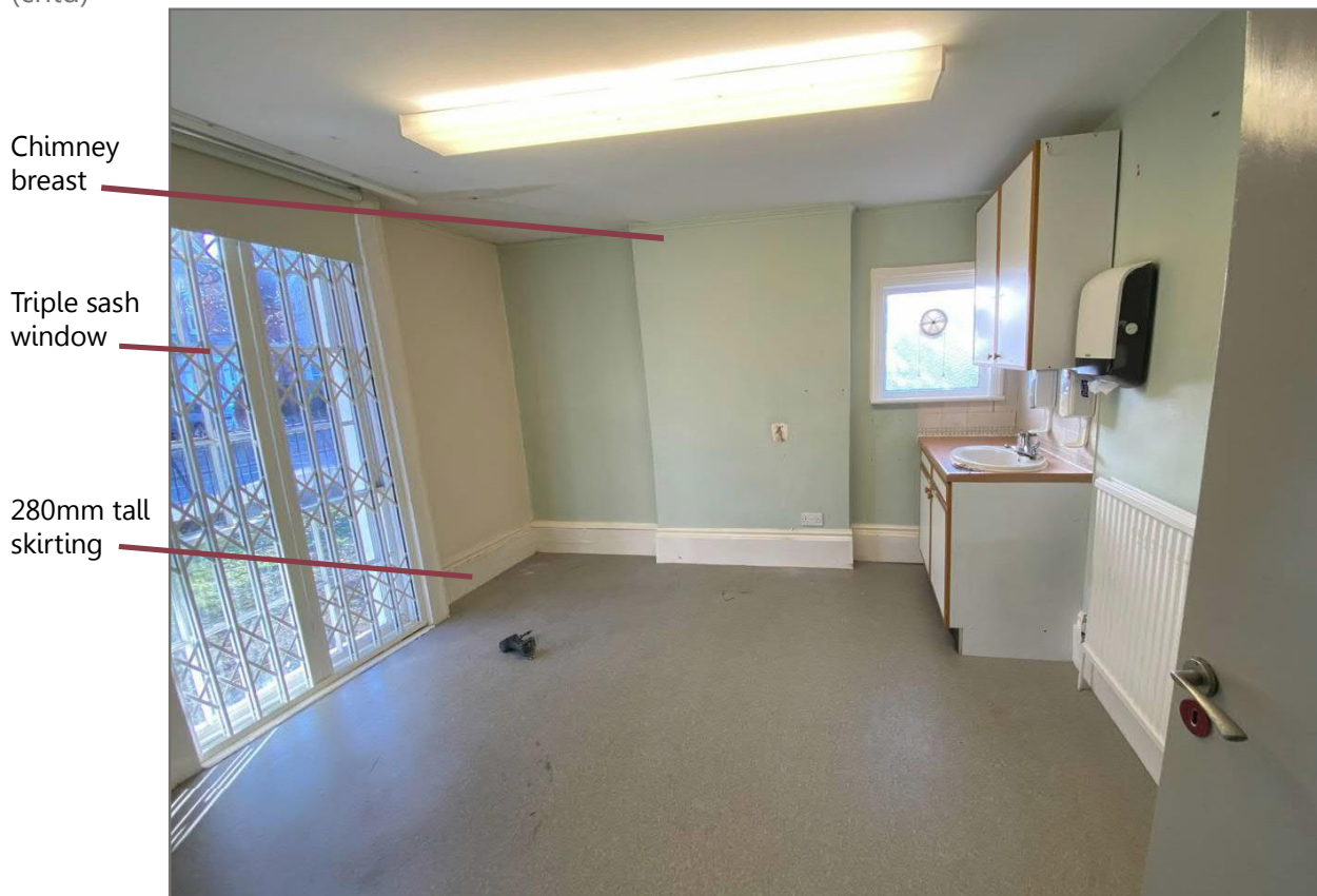
Image 31: Ground Floor west Reception Room (latterly a Consultation Room)
