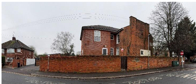
Picture 12: View from Highgrove Street
