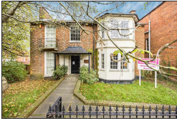
Picture 2: Front View
