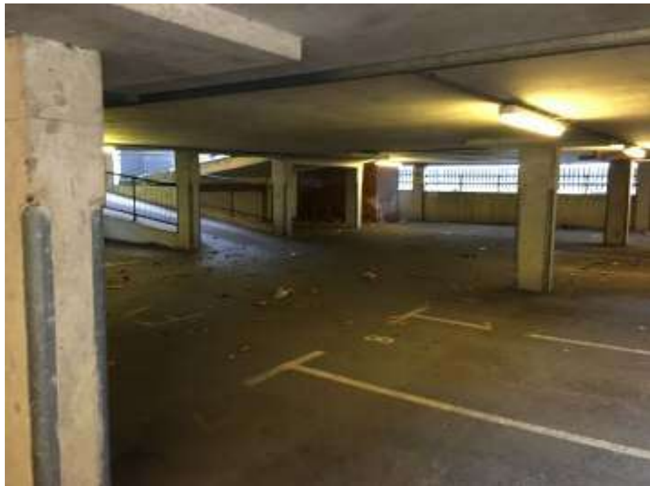
Photograph 4 Internal view of the multi-level car park
