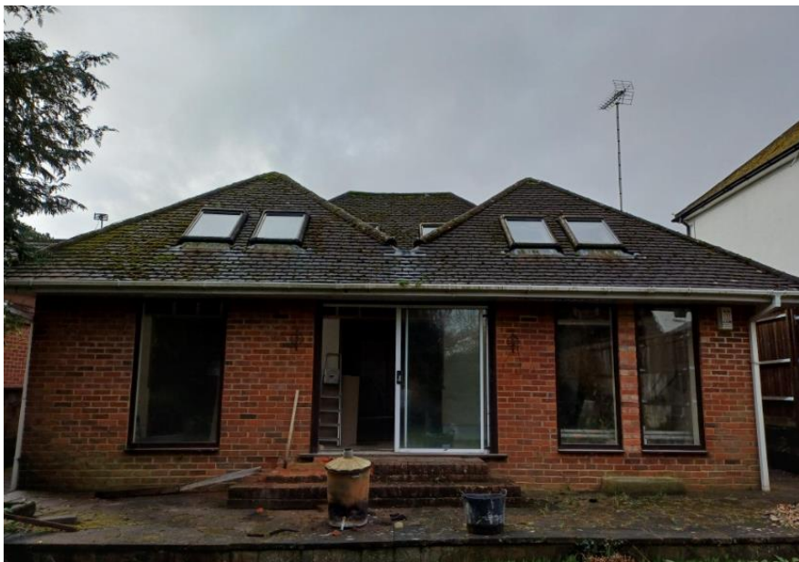
Figure 1 Rear elevation of the property. Image taken by planning officer on 6th February 2026.
