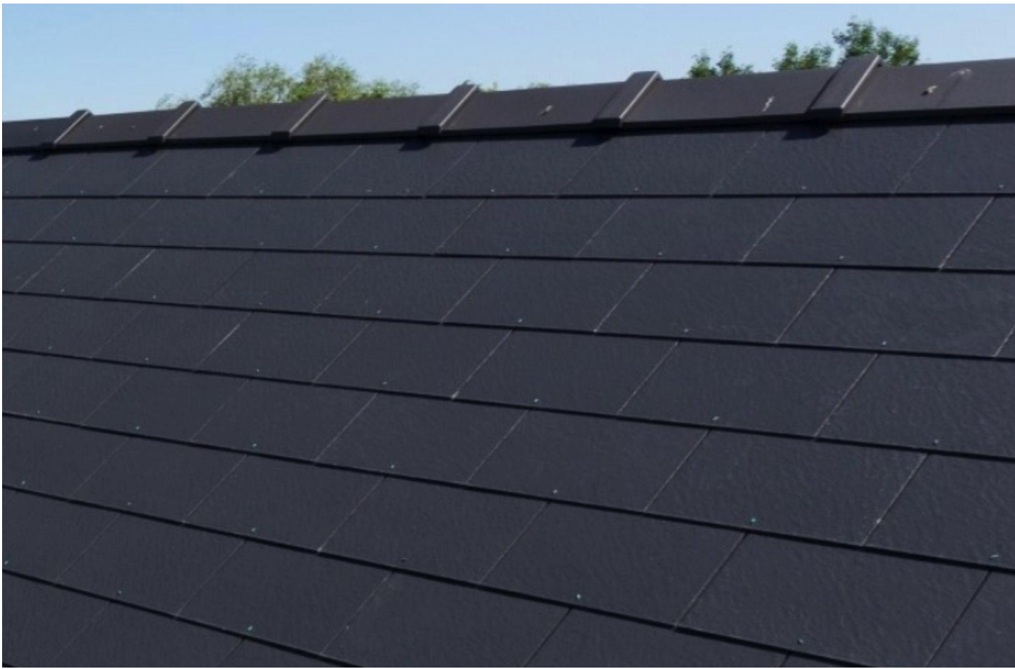
3 Marley Eternit - Cedral Thrutone Textured fibre cement slates
