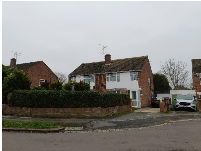
Fig 1: View from the front of 21 Riley Road (23/12/2025)
