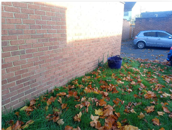
Fig 2.1: Trial Hole 2 Location
